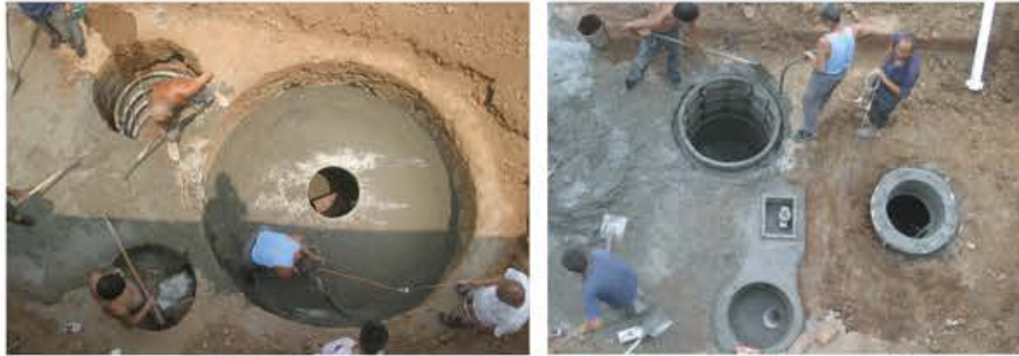
Construction of the Bio-gas tank in the backyard
