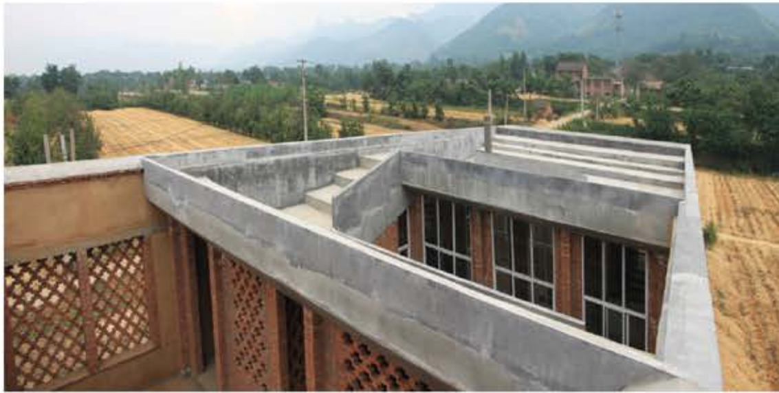
Stepped Roof of the House for Rainwater Collection
