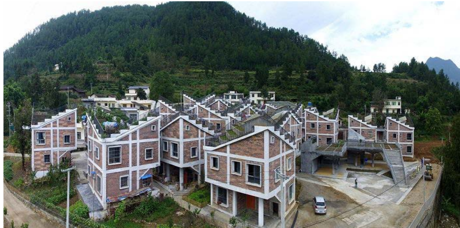
Stepped roof merged with the mountainous landscape
